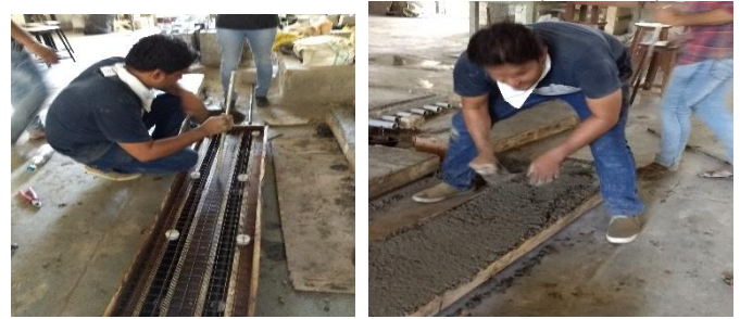
Fig 3 formwork preparation and castin
