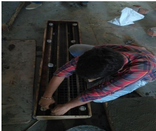
Fig formwork preparartion and castin
